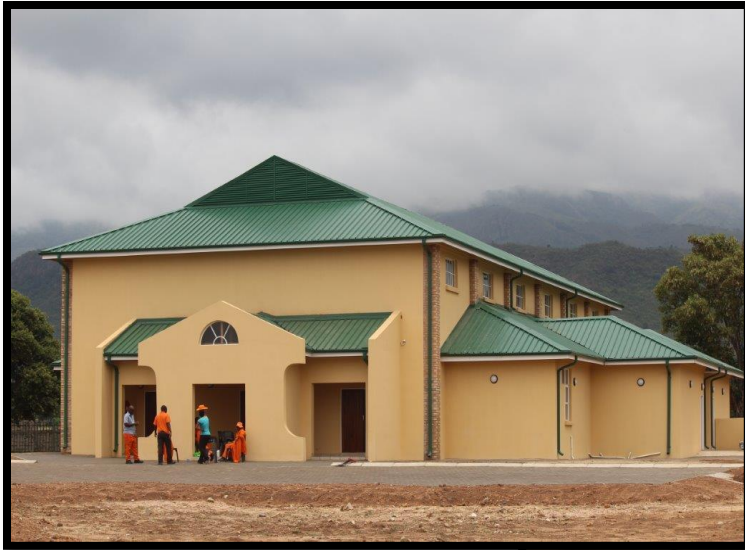
Moshate Community Hall
